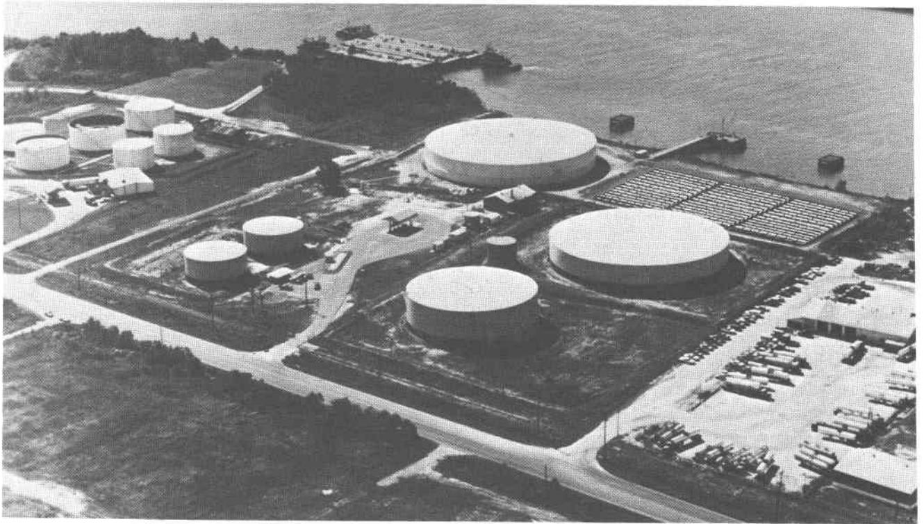
FIGURE 1. ERGON'S MOBILE BULK TERMINAL
