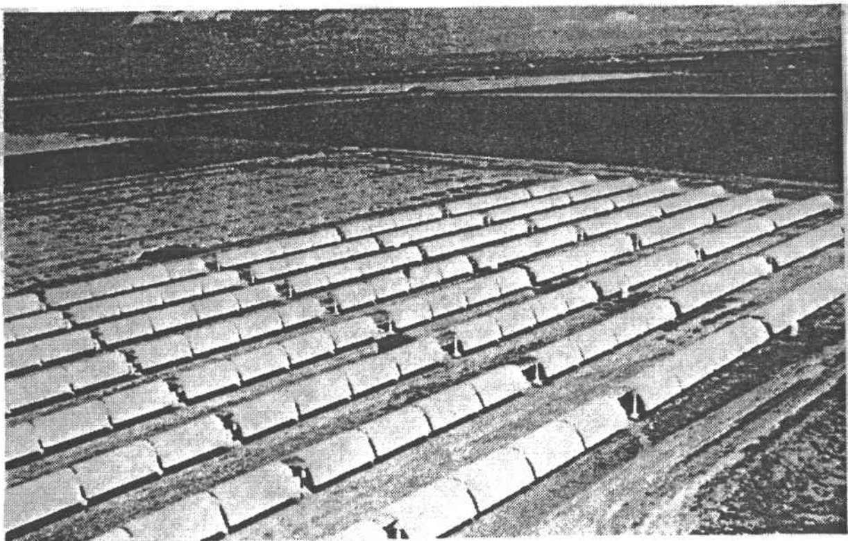
Figure 9. 150 kW Irrigation Pumping Experiment; Coolidge, AZ
