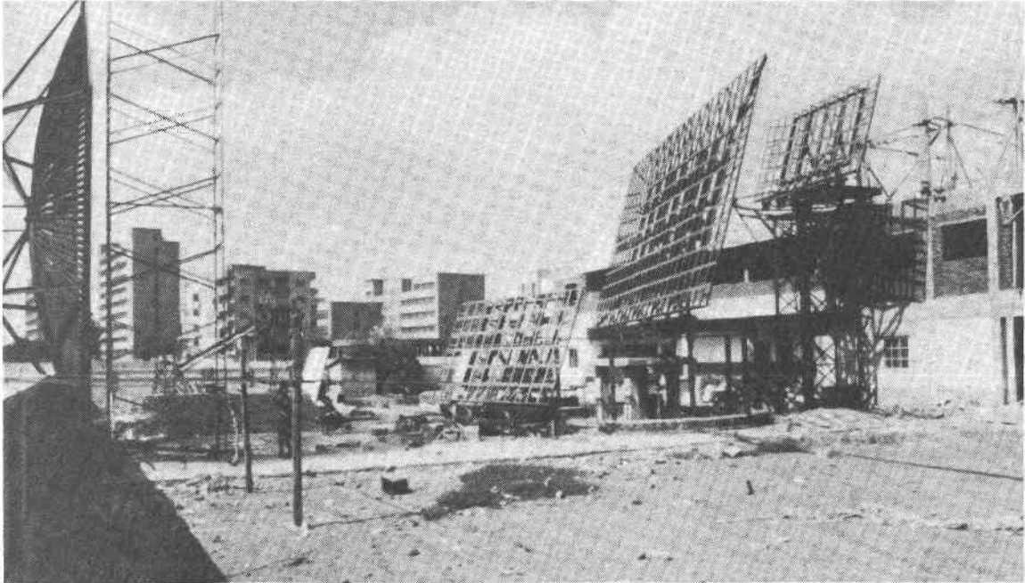
Figure 33. Construction of Solar Furnace Test Facility at National Research Center, Cairo, Egypt.
