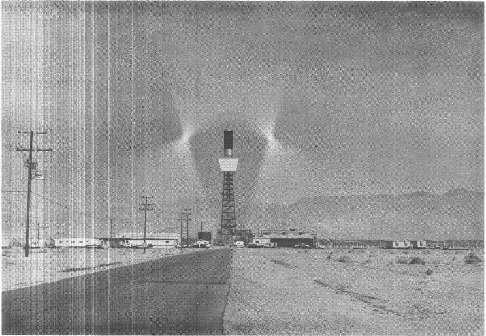
Figure 2.6. Receiver tower at Solar One showing luminous areas at standby focal points.
