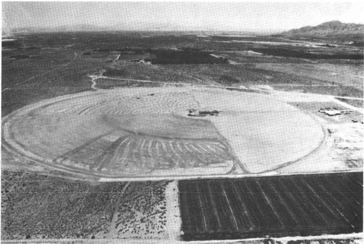
Figure 2.3. The Solar One site looking east across the heliostat field, Spring 1980. Work on heliostat pedestals has begun. Most ecological studies were conducted on the eastern sector downwind of the site between the periphery of the field and the agricultural land at top of the photo.
